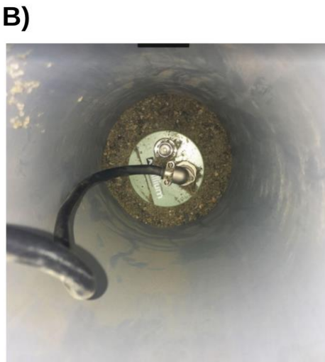
Figure 2. a) Example of the footprint of a single seismic monitoring station, showing solar power panels and the top of the short borehole containing the seismometer (Nanometrics Trilium T120). The digitizer (Nanometrics Taurus) and other electronics (e.g., cables, modem, etc.) are housed within the light grey box halfway up the solar panel pole. b) Example of the depth of borehole (~30 cm) containing the buried seismometer. Sensors were buried just below the surface to reduce surface noise (e.g., meteorological, traffic, etc.).
