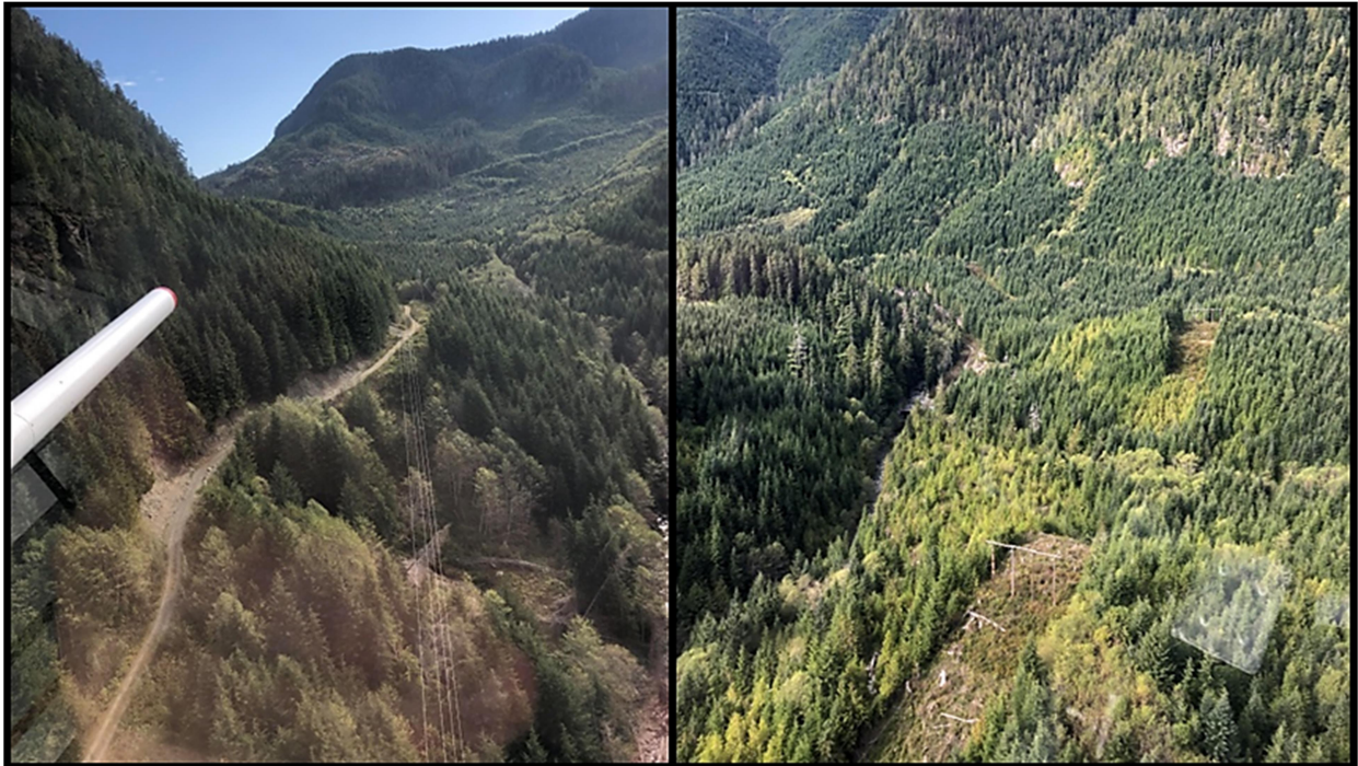
Figure 18: Examples of valley-spanning powerline northwest of Tahsis that resulted in height deviations.
