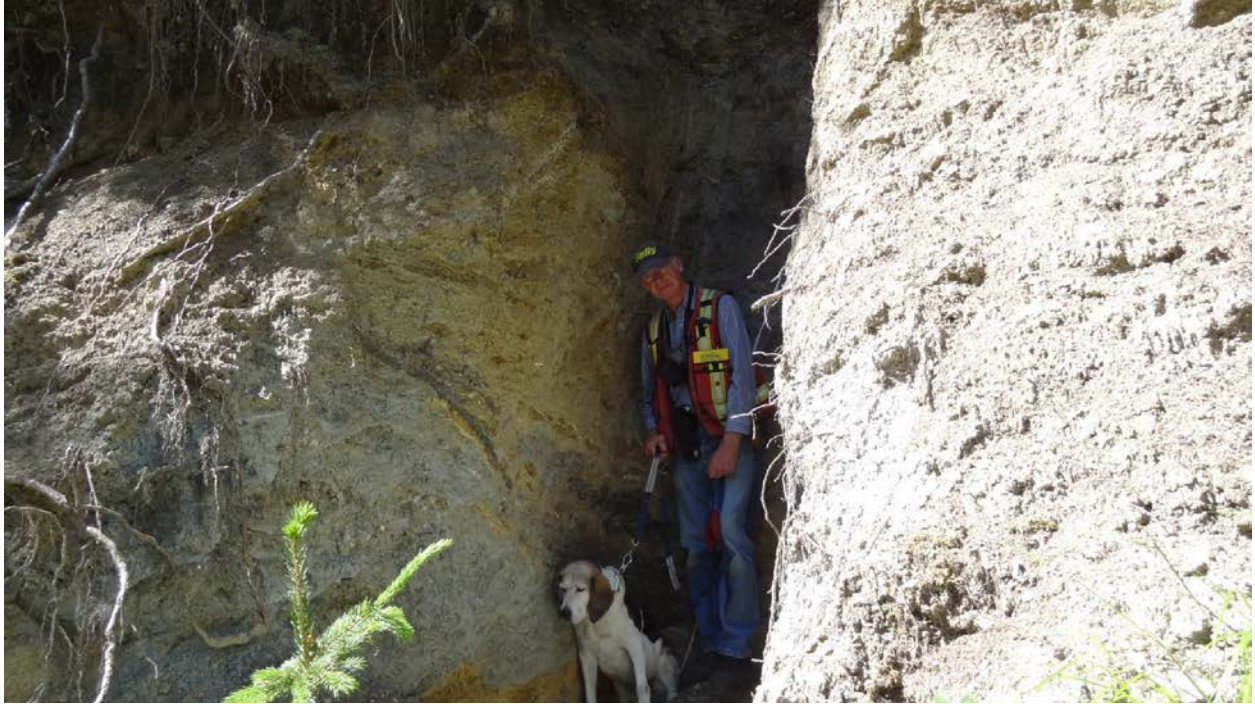
Photo 3. LANF on Estella Ridge. UTM 11 600554 5517580, elevation 1575. Three metre portion of LANF exposed in road cut. Fault material is incohesive gouge of rock flour and chips with about 10% rock fragments to 5 cm. Planar alignment of the gouge is 20°-258°.
