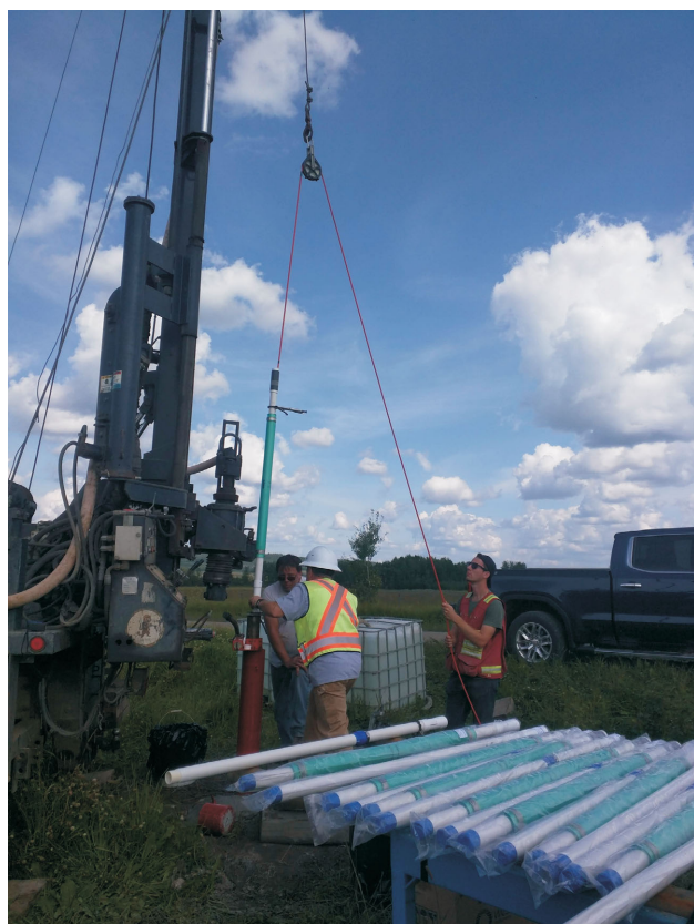
Figure 4. Installation of Westbay Instruments system in well EERI-11. The foreground shows the layout of the packers (green) and casing with measurement and pumping ports (white casing) during installation.
