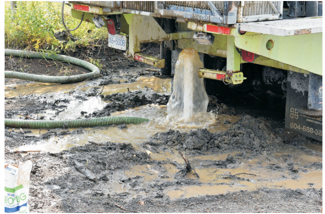
Figure 8. Artesian well flowing (approximately 22.5–45 L/min) after completion at Groundbirch field, Peace region, British Columbia. The well was immediately and temporarily sealed with a polyvinyl chloride (PVC) end cap and subsequently permanently sealed with a subfrost artesian packer with built-in sampling valve during a follow-up fieldwork campaign.
