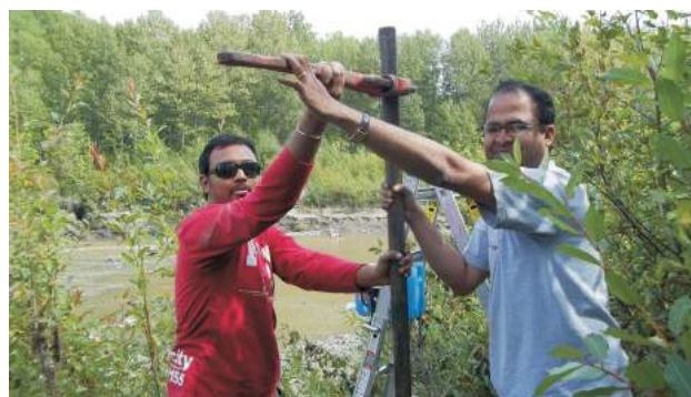
Figure 4. Stages of piezometer installation in the Mainstem sub-basin, Kiskatinaw River watershed.
