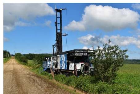
Installation of a groundwater monitoring well
