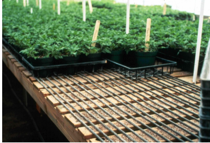
Figure 43. Bench top plastic tube heating system (site visit Lund, 2002).
