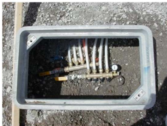
Figure 49. Details of the header pipe with PEX pipe for a pavement snow melting system (Boyd, 2003).
