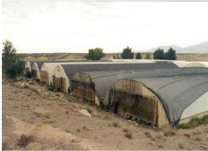
Figure 40. Arched greenhouses with cover for solar reduction (New Mexico, USA) (Witcher and Lund, 2002).
