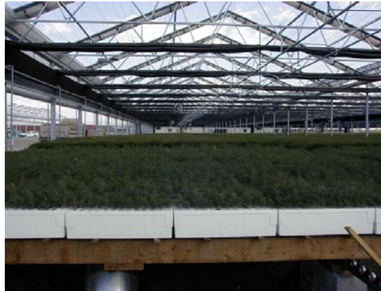
Figure 44. IFA Greenhouses in Klamath Falls, Oregon, USA, growing tree seedlings. Note overhead sprinklers. Heating system is under bench forced air (Geo-Heat Center site visit, 2002).
