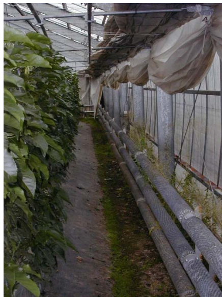
Figure 42. Finned tube heat pipes along the greenhouse outer wall (site visit Lund, 2003).
