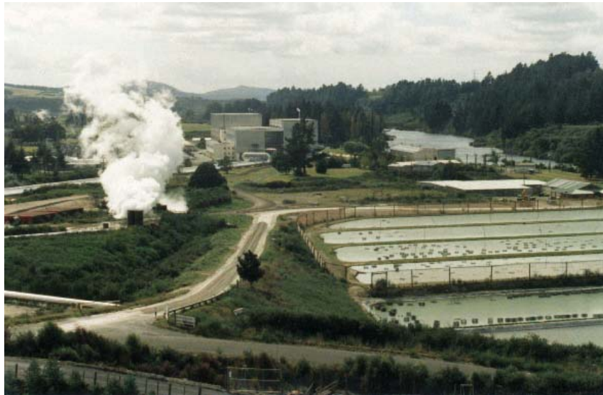
Figure 29. Wairakei, New Zealand, commercial Malaysian prawn raising facility, using waste water from a geothermal power plant (Lund and Klein, 1995).
