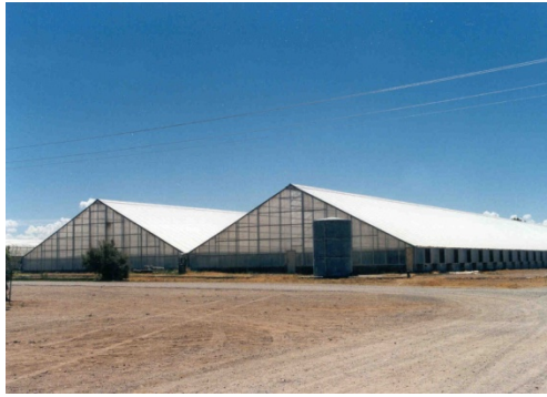
Figure 37. Greenhouses with steep roofs used in areas of heavy snowfall (New Mexico, USA) (Witcher et al., 2002a).
