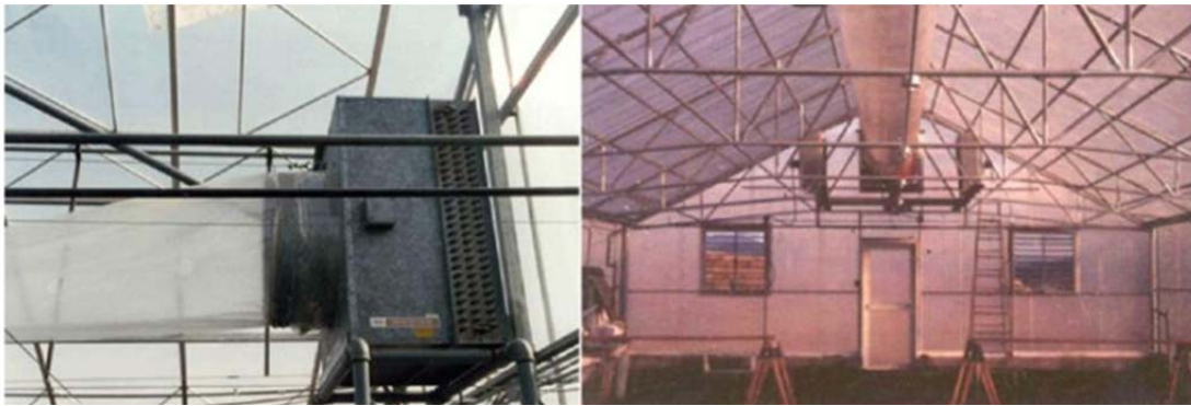
Figure 41. Forced air heating system with overhead plastic tubing perforated along the bottom for the air flow (Witcher et al., 2002)(site visit Lund, 1977).
